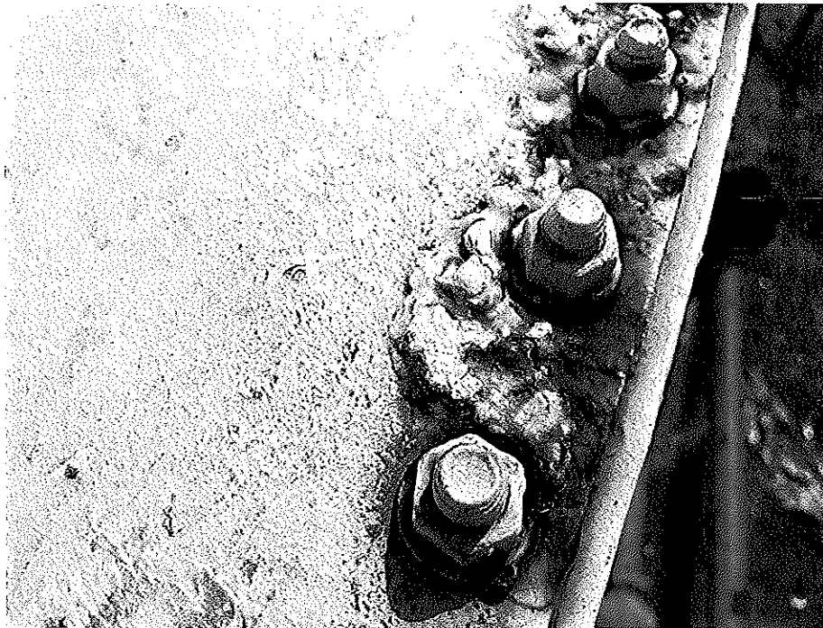
Photograph 12: Moderate corrosion on the outside roof bolted connections
