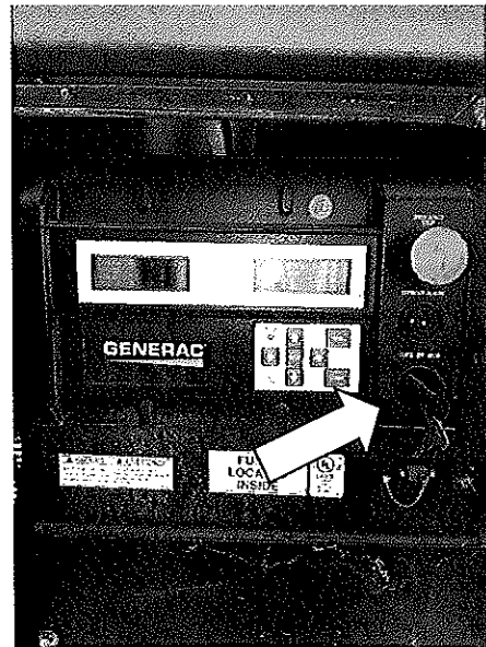
Figure III– Turn switch to start to operate generator and turn off to shut down generator.
