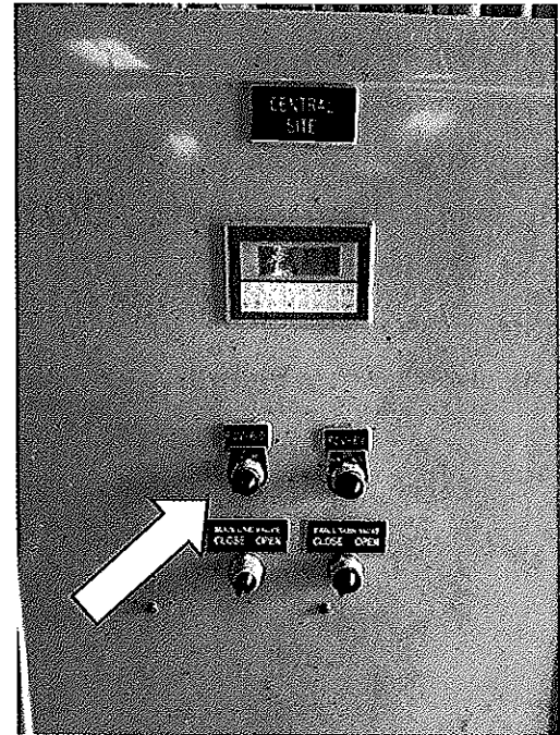
Figure VII – Turn switches to off before opening the M.O.V. manually. Back to auto after Ground Storage tanks are at desired levels.
