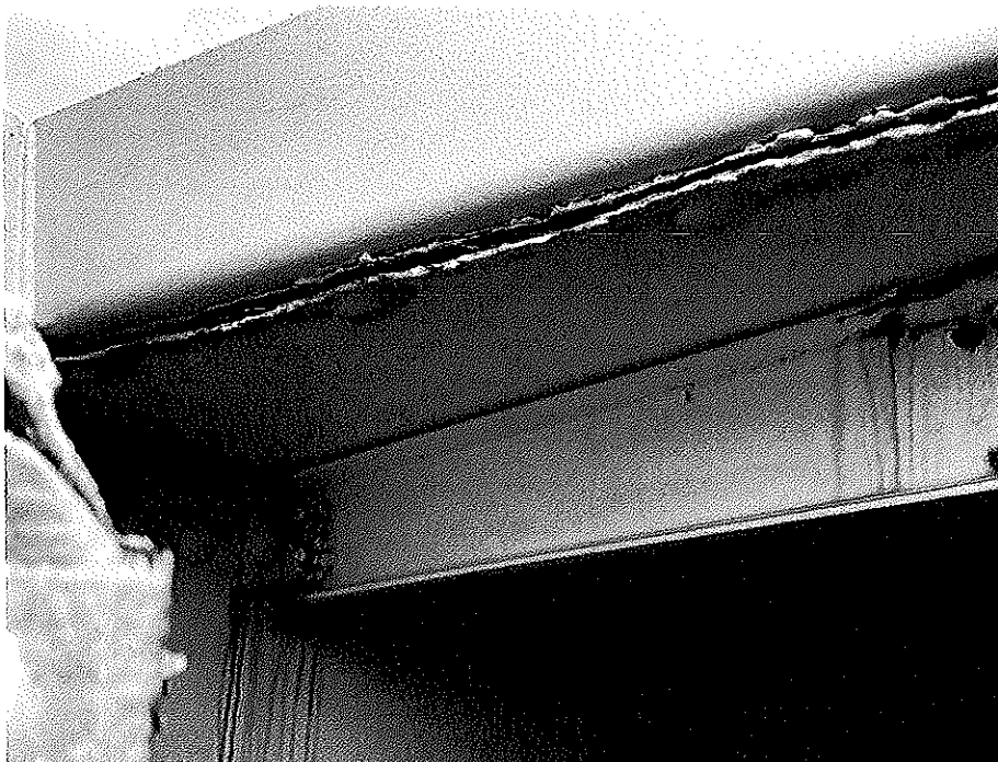
Photograph 14: Moderate corrosion on roof shell, roof framing and severe corrosion at bolted connections
