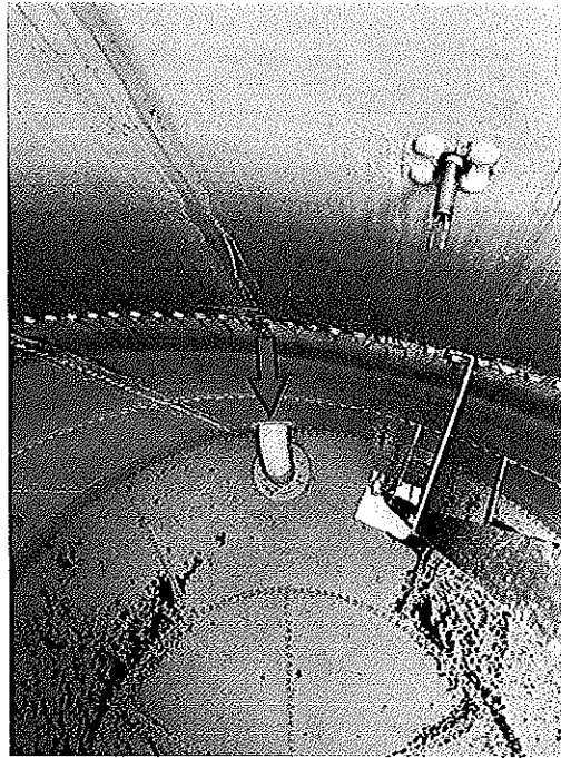
Photograph 17: Tank water outlet inside view looking west
