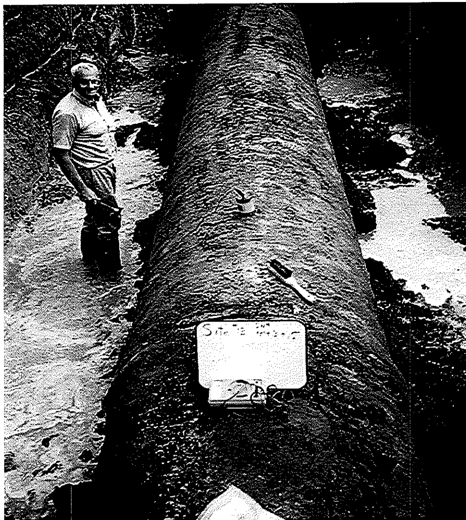
Figure 8. Excavation 11 - Pipe Joint Pitting.
